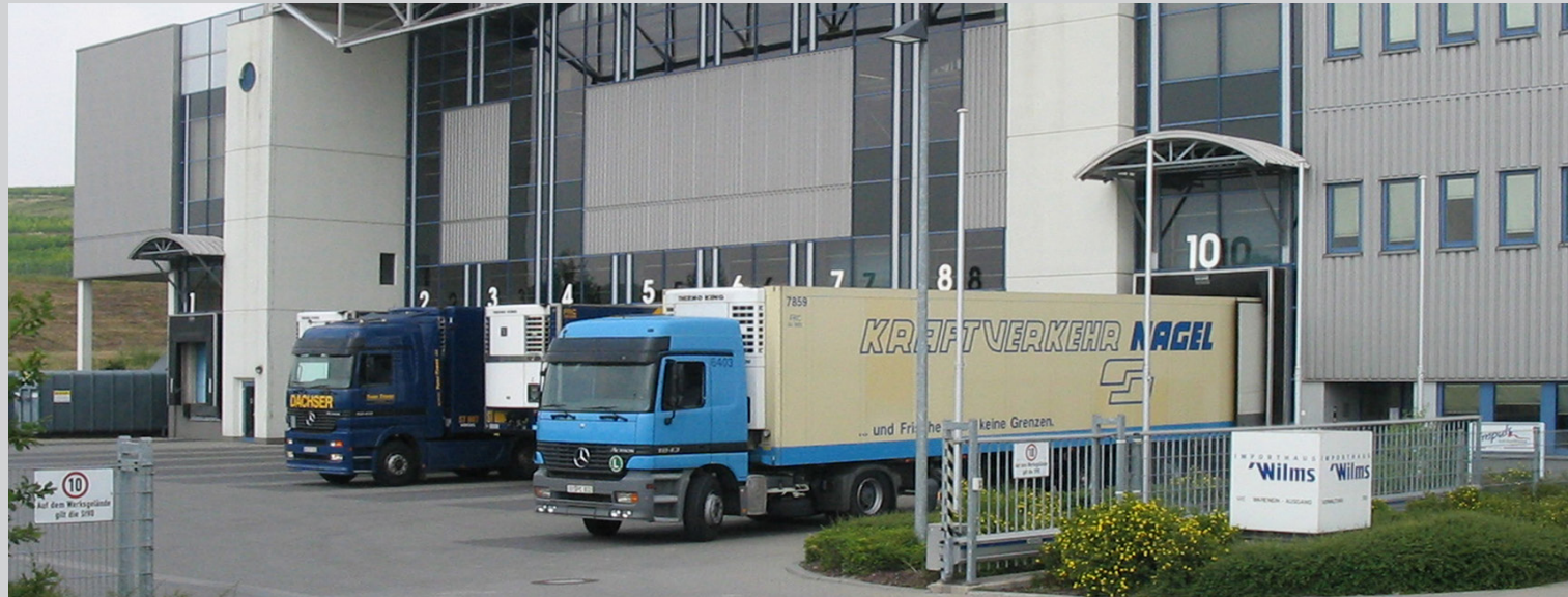
View of the distribution centre in Alzey
